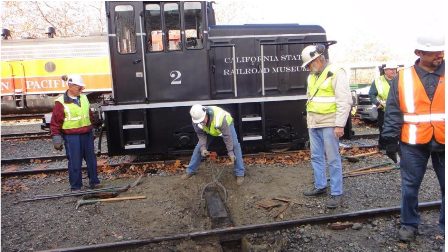
After the 125 pulled a tie out, Steve grabs it with the tie-tongs to get it out of the way for disposal
