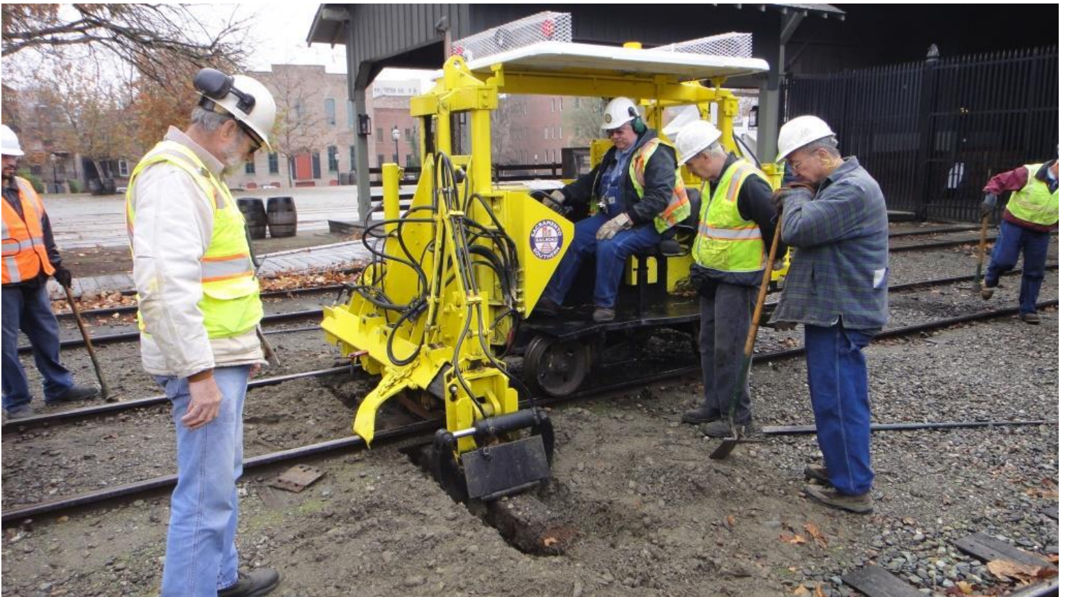
With the trench dug, Chris pulls the tie out
