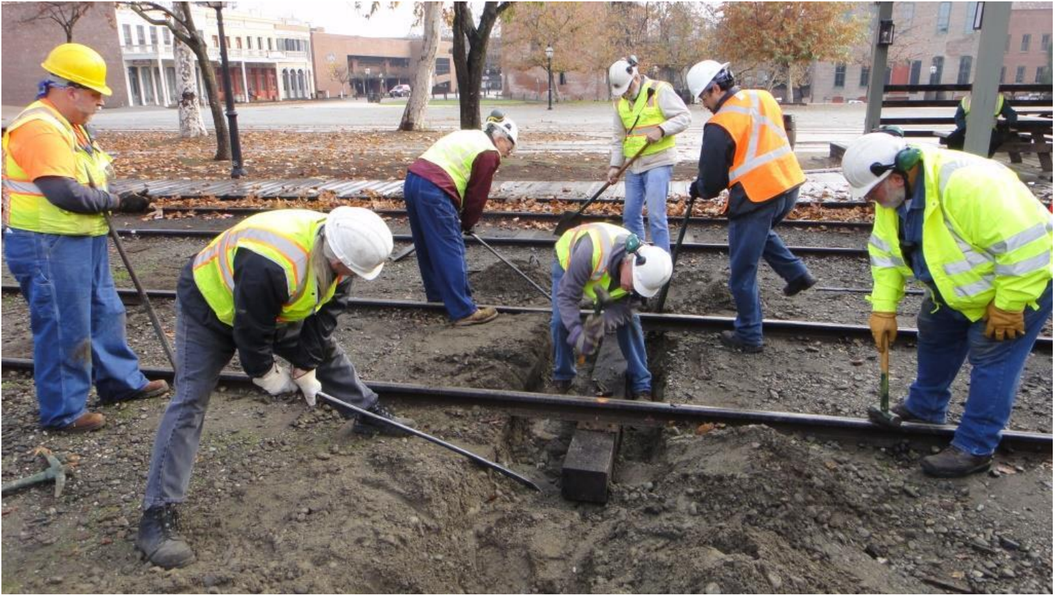
With a new tie in place, Steve and Frank set spikes, Fred and Clem nip it up, while Mike F., Alan, and Jose back-fill the crib
