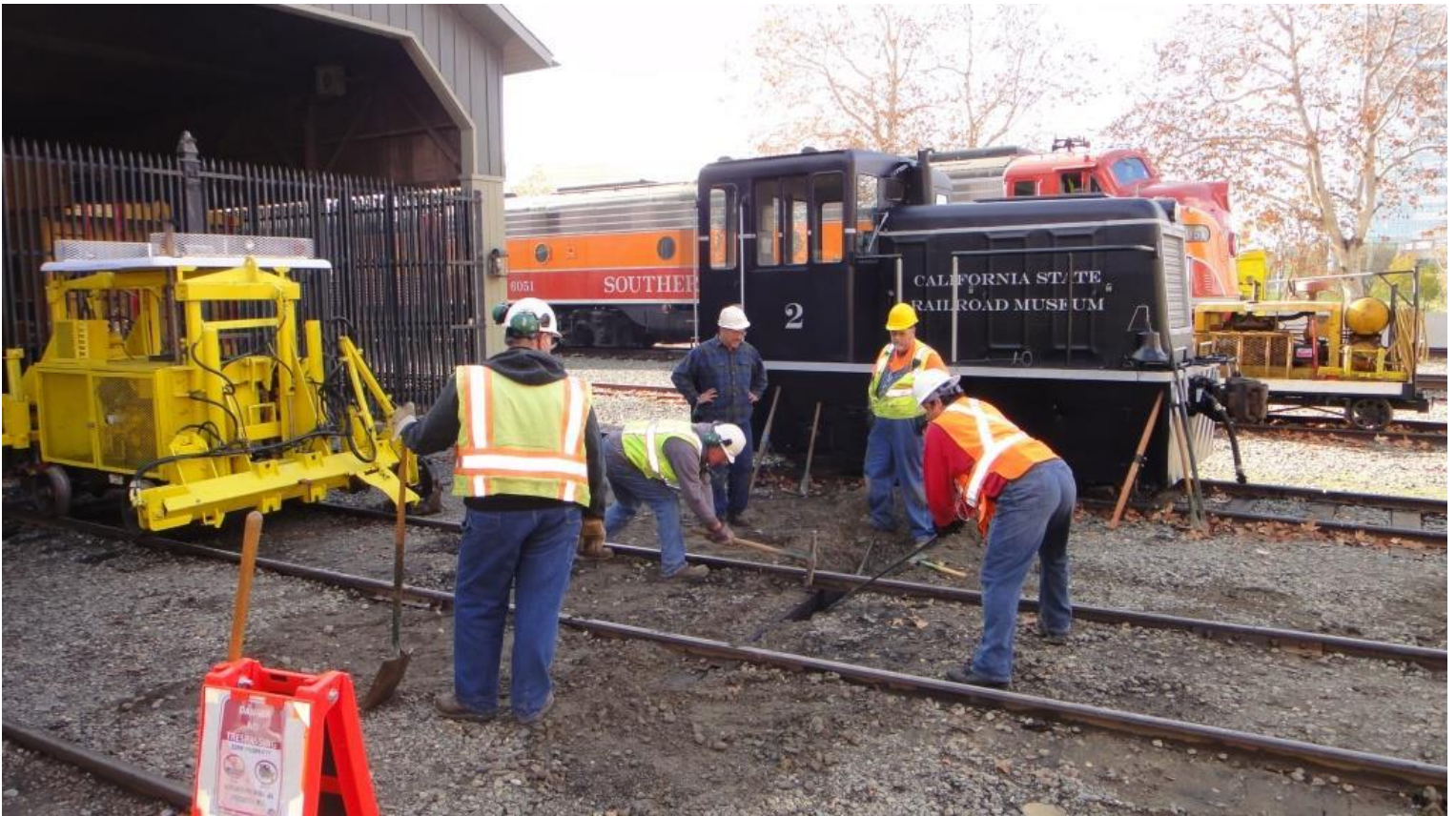
Jose nips-up the tie while Steve drives the spikes
