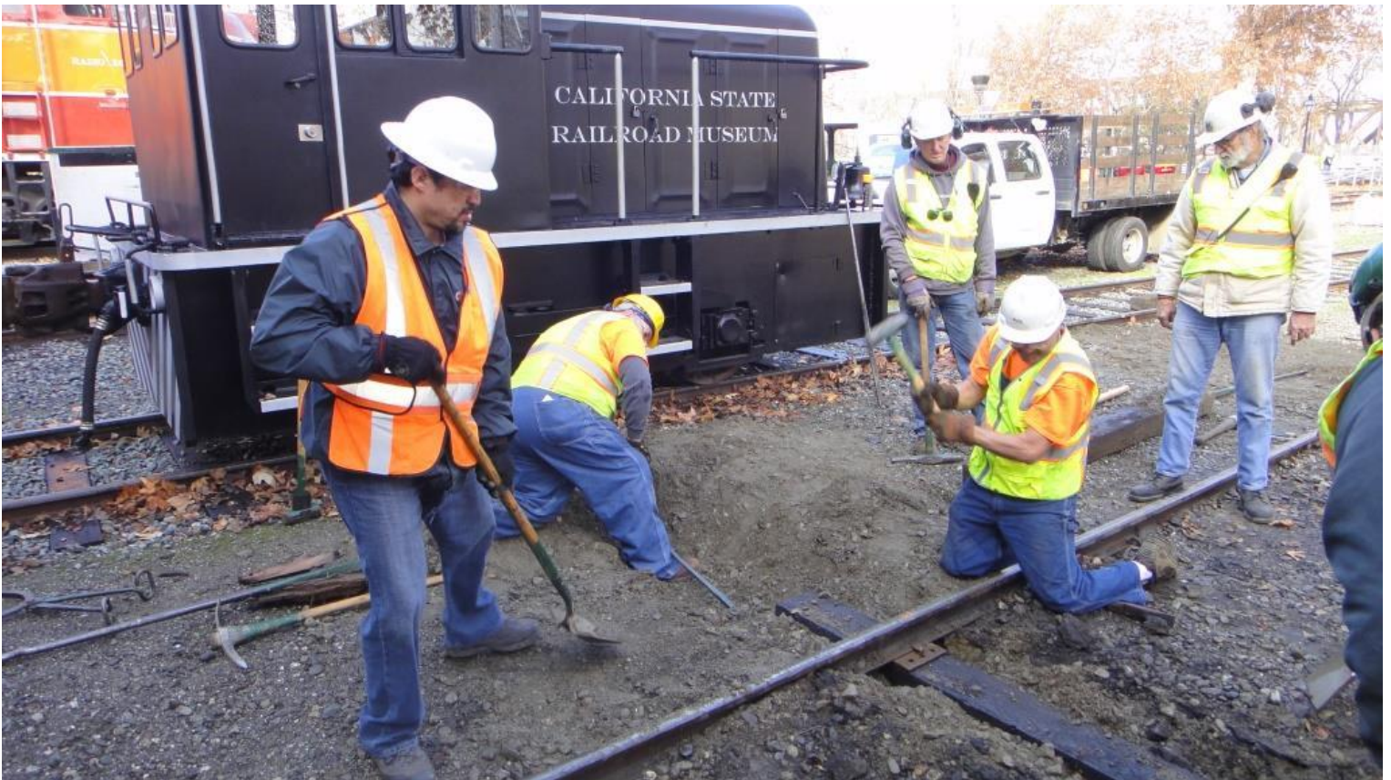
Jose back-fills the tie-crib while Mike F. nips-up the tie as John drives a spike with a short-handled sledge
