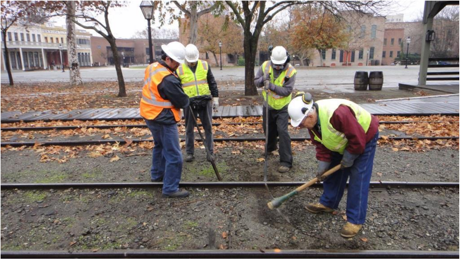
Jose, Fred, Steve, and Clem start digging out the ties and pulling spikes along Track 2
