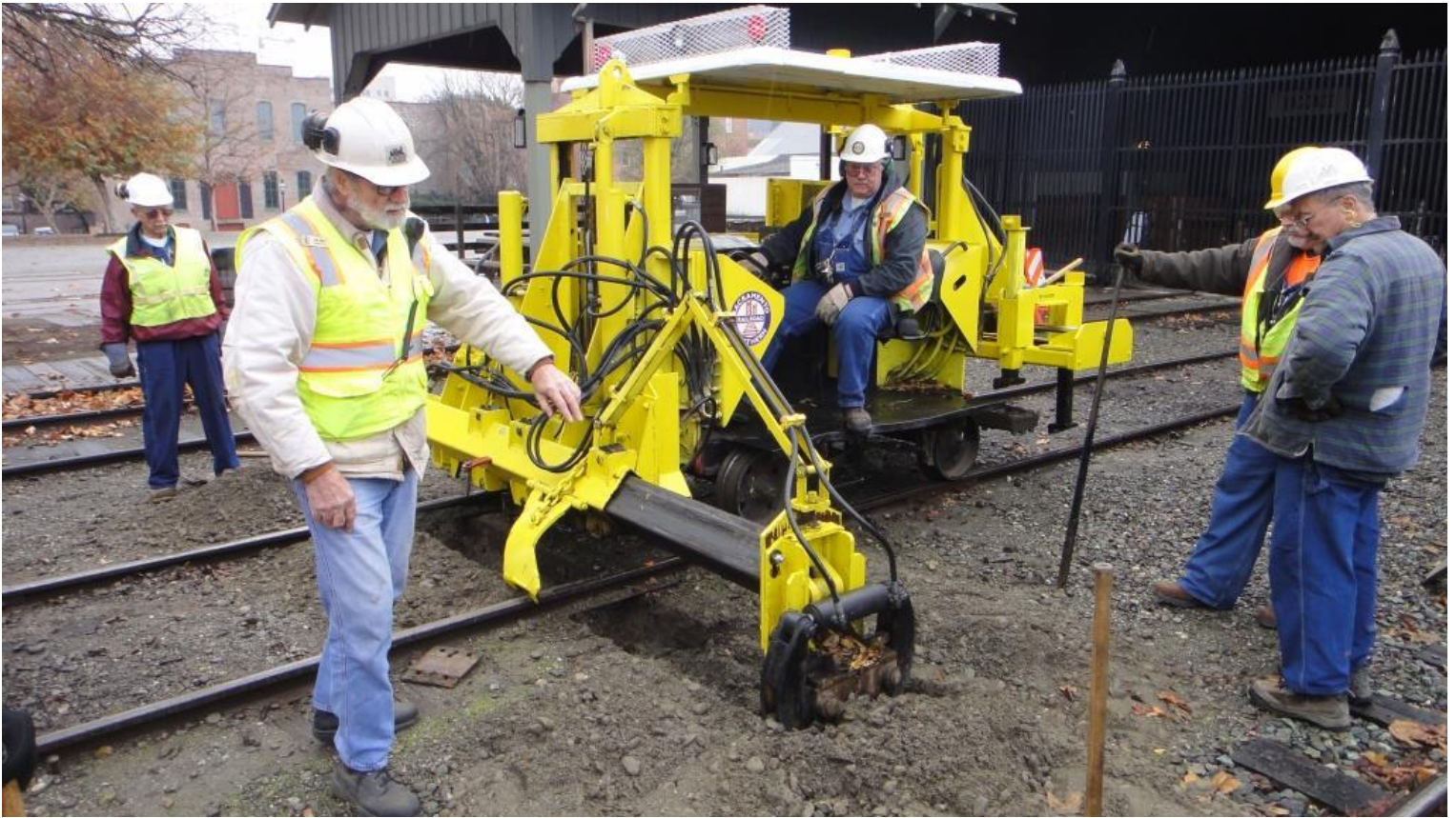
Chris on the Jackson 125 tie-exchanger uses the trenching feature to create a hole big enough for the old tie come out and new tie to go in
